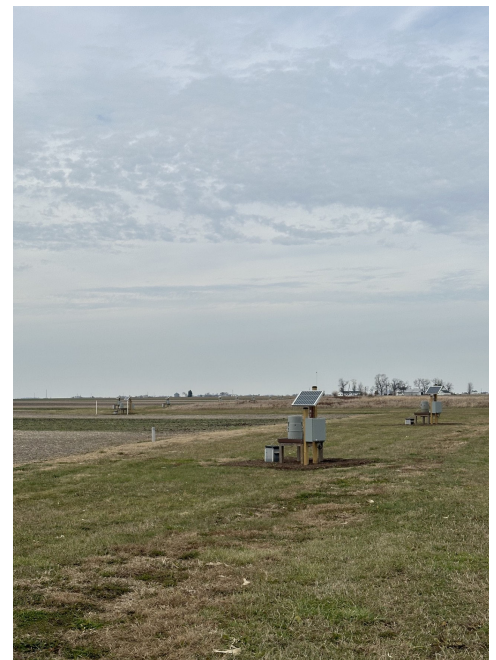
Eric’s tile gauging stations installed along a filter strip.
